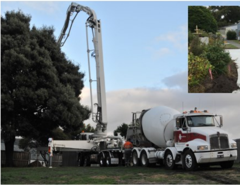
Hazell Bros concrete being pumped over the trees onto the pathways.
