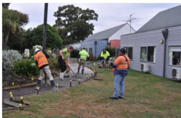
Designing the pathways. Pumping concrete for the paths Boxing the paths.
