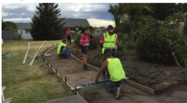
Designing the pathways. Pumping concrete for the paths Boxing the paths.
