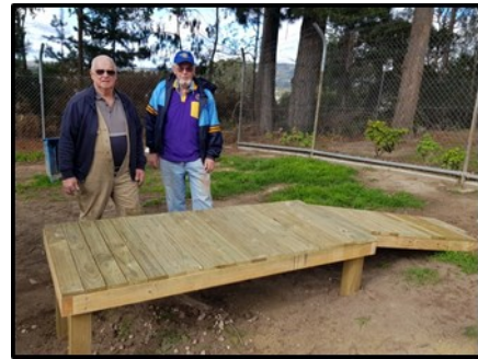
Right: Noel & Vere with a finished platform
